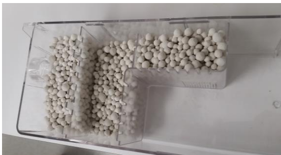
Figure 1: Evenly fill first three chambers of the tank with neutralizer media
